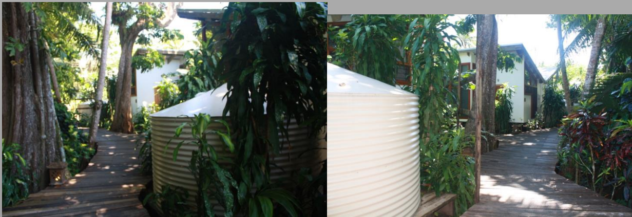
RAINWATER TANKS OUTSIDE EACH RESORT ROOM
