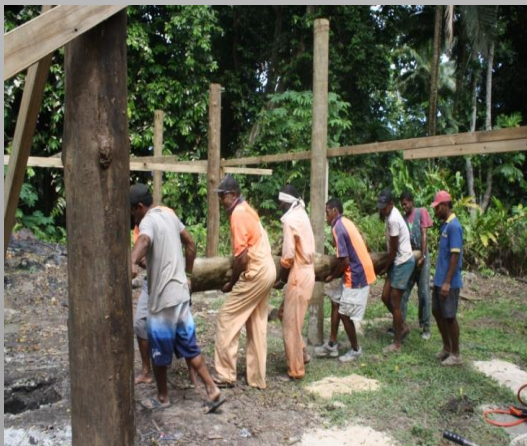
STAFF CONSTRUCTING THE YOGA CENTRE
